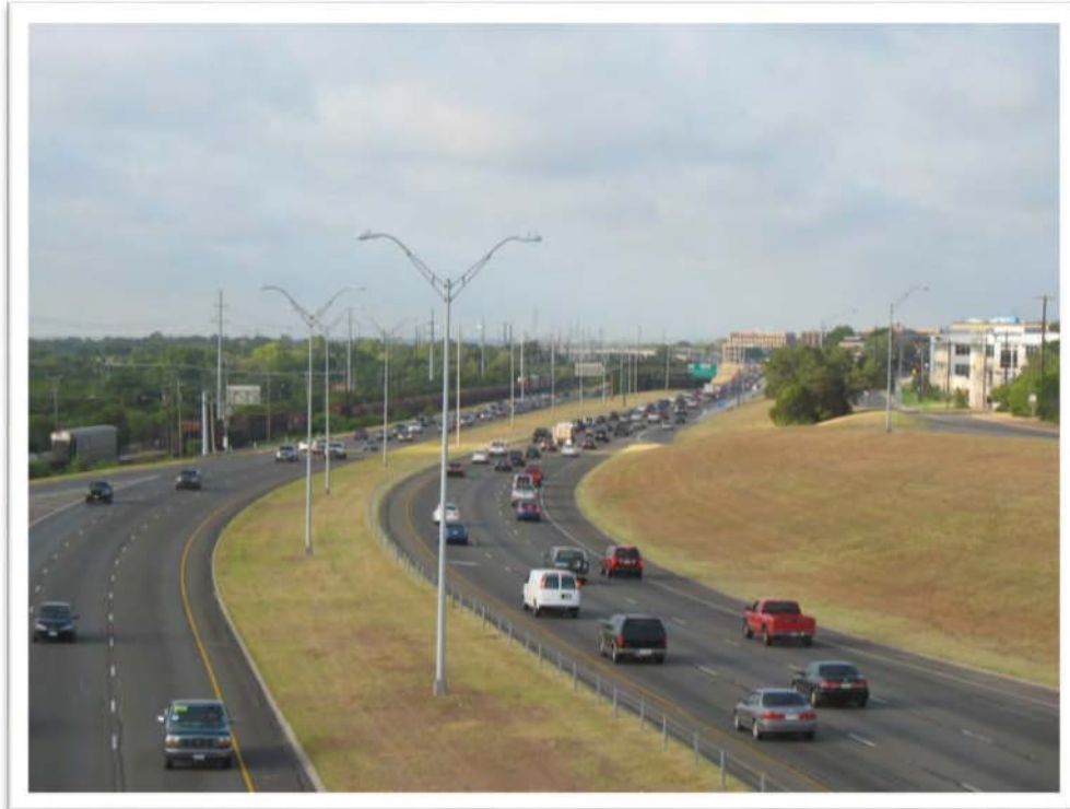
Photo 11: Photo taken from the Far West Boulevard bridge looking south on MoPac.
