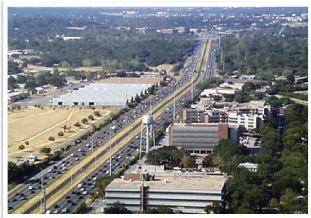
Photo 2: MoPac facing north near 35 th Street. Camp Mabry is on the left (west) side of the highway.
