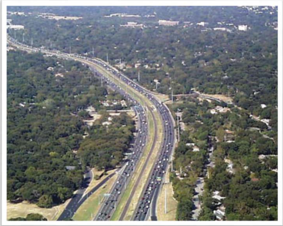
Photo 3: MoPac looking south near Windsor Road.
