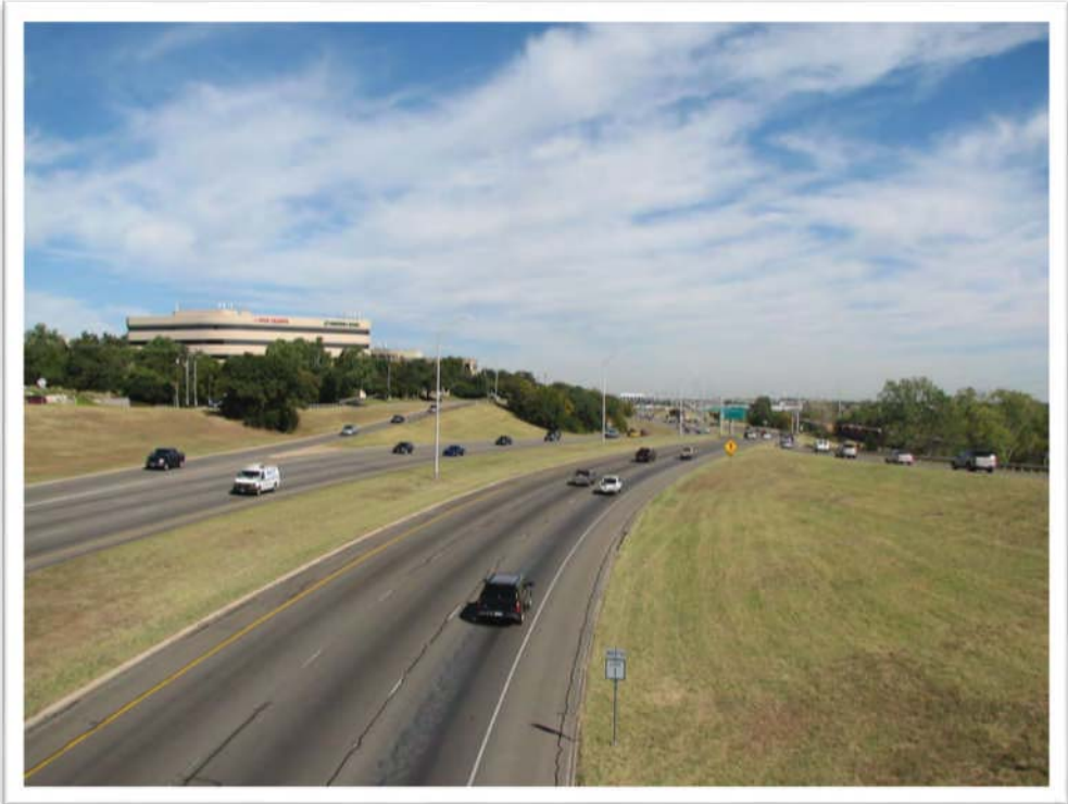
Photo 10: Photo taken from the Far West Boulevard bridge looking north on MoPac.
