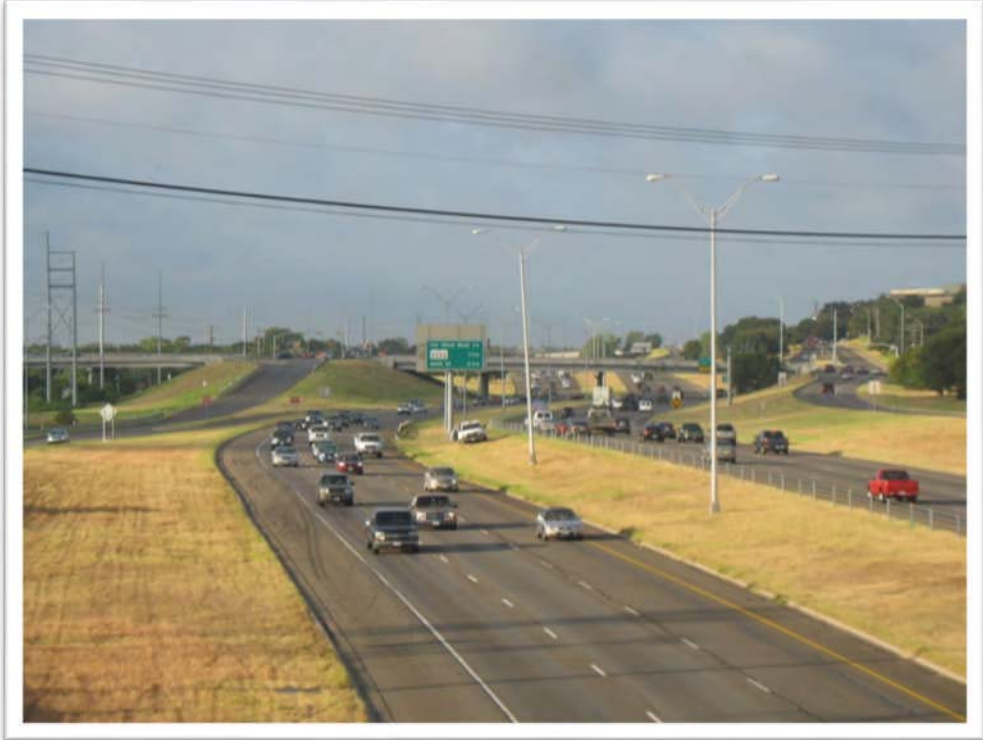
Photo 9: Photo taken from the Steck Avenue bridge looking south on MoPac.
