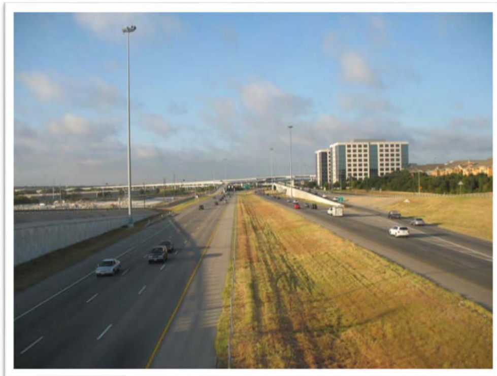
Photo 6: Photo taken from the Loop 360/Capital of Texas Highway bridge looking south on MoPac.
