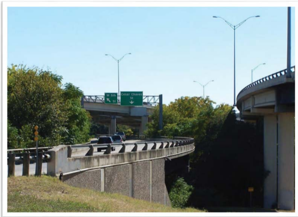
Photo 14: Looking south along the MoPac exit to Cesar Chavez Street/5 th Street. The structure to the right is the on-ramp connecting Winsted Lane to southbound MoPac.
